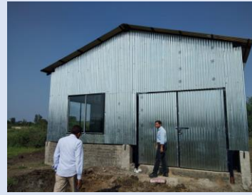
Setting up waste management shed
